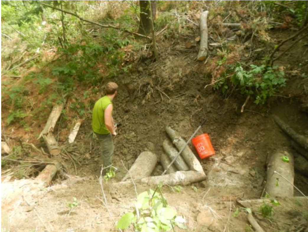
Figure 2. Gully restoration using on-site woody vegetation
