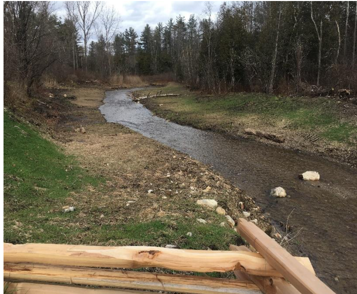
Photo: Reconnected Floodplain Along Tenney Brook at the Former Site of Dunklee Pond
