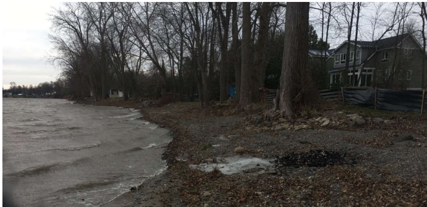
Photo 1: Area of erosion along the lakeshore
