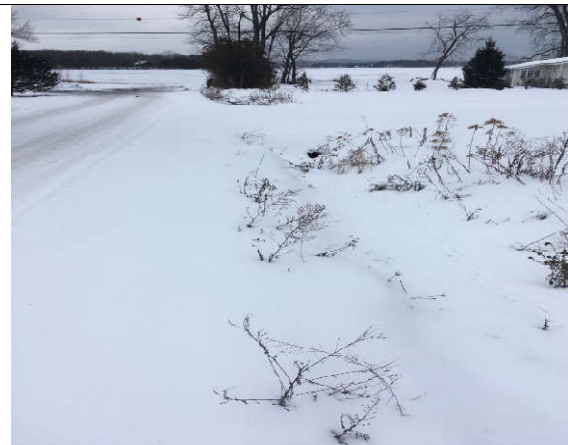
Photo 2: Driveway culvert in the ditch at the parking lot entrance
