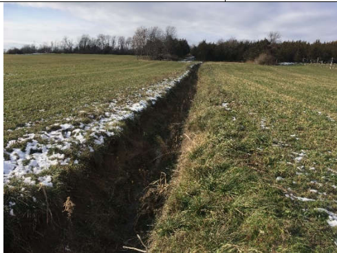
Photo 1: Incised ditched channel
