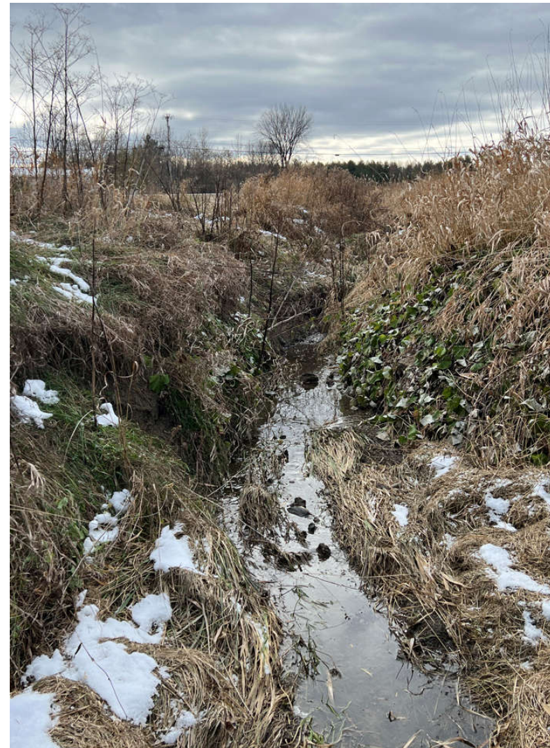
Figure 8: Eroded channel and headcut at the South Hero village center complex. The concept design for this area describes BMPs that would stabilize erosion and create floodplain access.
