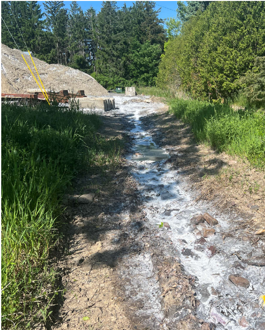
Figure 7: Runoff from the sand/salt pile at the South Hero Town Garage. The concept design for this area describes BMPs that would slow and treat stormwater runoff.
