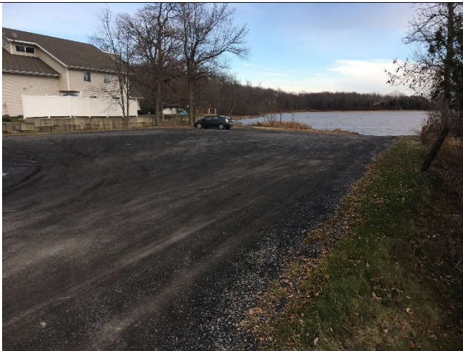
Photo 1: Boat launch with swale along the right side
