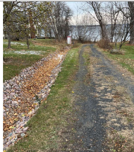
Photo 2: Stable ditch above ramp
