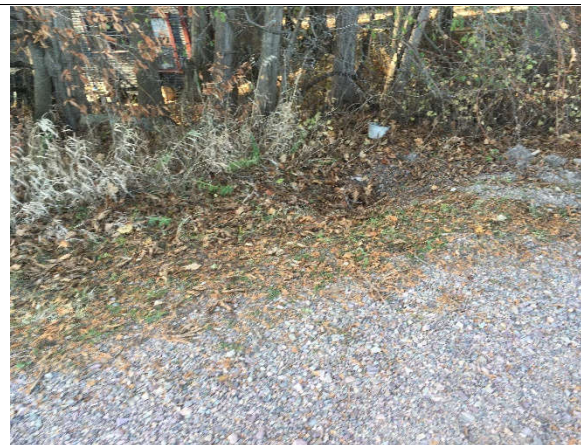
Photo 2: Forested area south of the driveway with existing culvert outlet.
