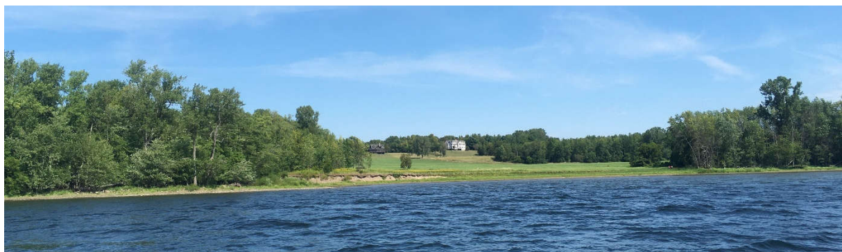
Photo 1: Area of erosion and lawn along the lakeshore
